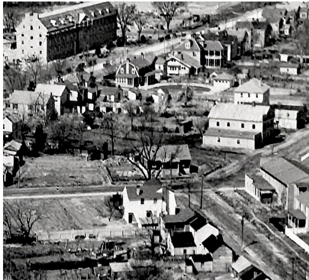
Digges House, between 1924-26, on its original site. Gambrel roof added along with two-story rear wing. In 1930 it would be moved a half block to the nw a located between the 2-story frame house and the pyramidal roof frame house in the upper right-hand corner of the photograph.
