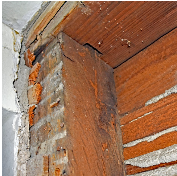
sw corner post tenoned into the plate
