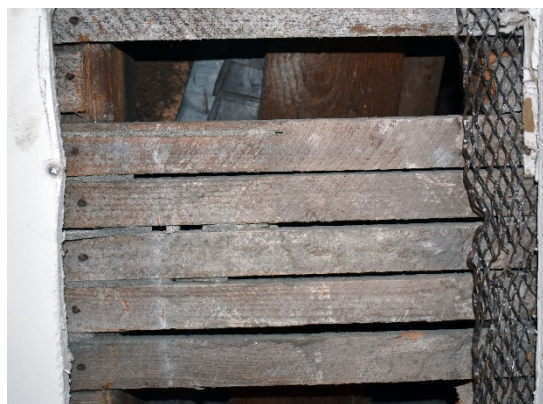
Circular sawn lath, secured by wire nails, c. 1924.
