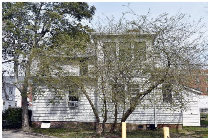
South end of house; two-story central block and one-story section to the right built on this site by the college between 1930-1933; one-story section to left added in the late 1930s or early 1940s.
