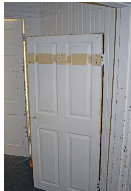
Reused 4-panel door, perhaps original stair closet, reset in vestibule in 1920s.
